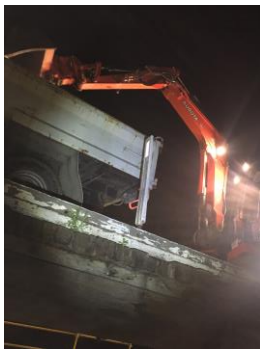
Left: Removal of bridge deck by excavator
